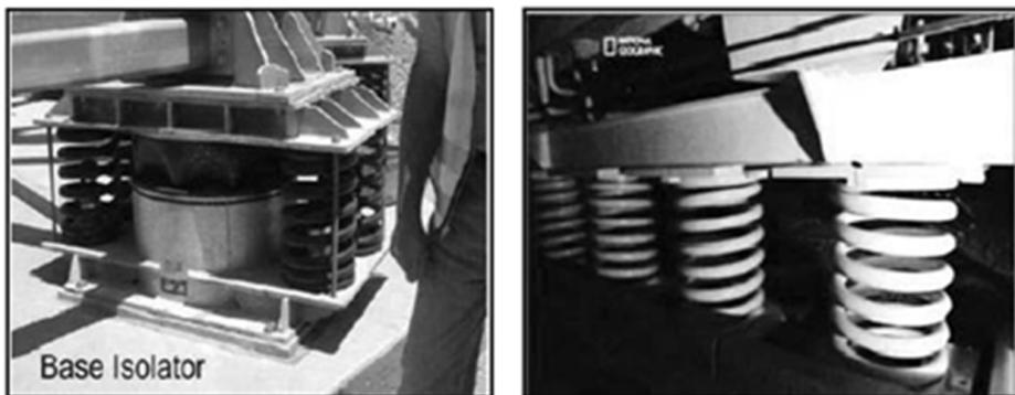
Fig. 16. A view of the damper springs at NORAD control and command center (Alhamad, 1996)
